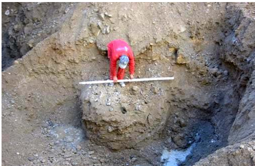
▲ Campo Prove : colonna Soilcrete Jet-Grouting
