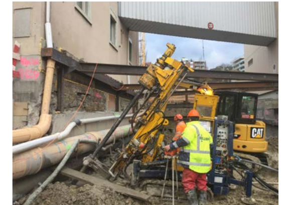
Underpinning works under limited space on site
