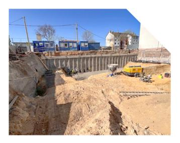
The project site itself was highly restrictive: a 35 x 25-metre inner courtyard accessed only through a single three-metrewide passage. Every delivery, machine, and material had to pass through this bottleneck, requiring meticulous coordination. Even the slurry pit for jet grouting had to be downsized due to soil handling and logistics.
