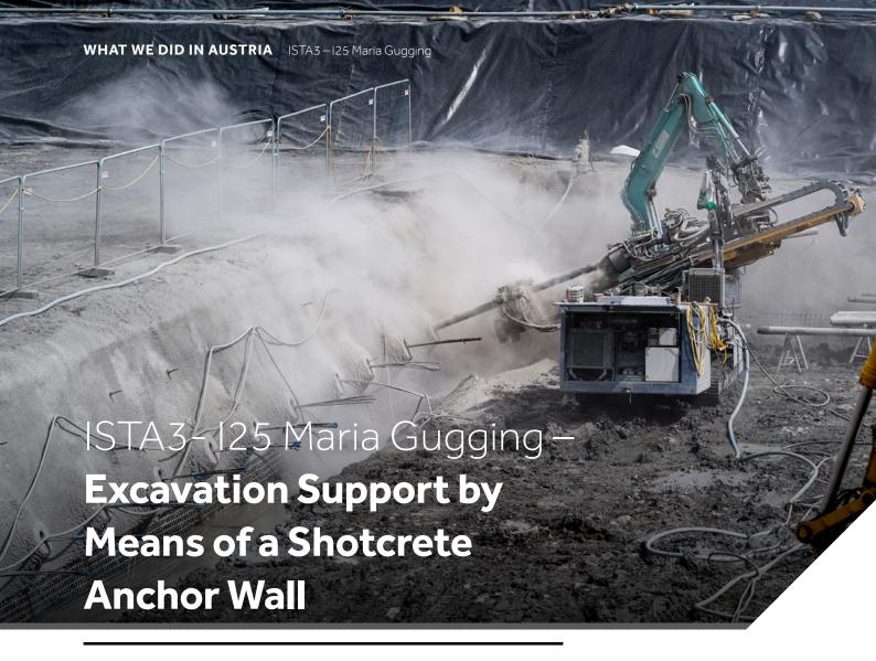
In the heart of the Vienna Woods, the Institute of Science and Technology Austria (ISTA) continues to expand with the construction of the new I25 building. The project requires extensive special foundation works, including an excavation pit down to 38 metres deep, supported by anchor walls, bored piles, and soil nail walls.
