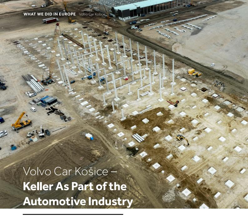
The construction site is located in the Košice district, approximately 12 km south of the city of Košice and west of the village of Valaliky. For the automotive company Volvo, it was necessary to establish several halls over an area of approximately 300,000m². Due to the geological conditions, deep foundation using large-diameter piles was chosen. Upon completion, the individual halls will be used for the production of Volvo cars
