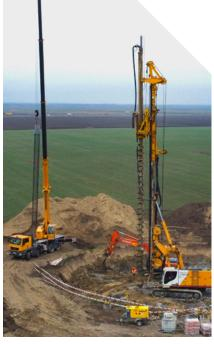
**CONSTRUCTION OF CFA PILES** with the BG36
