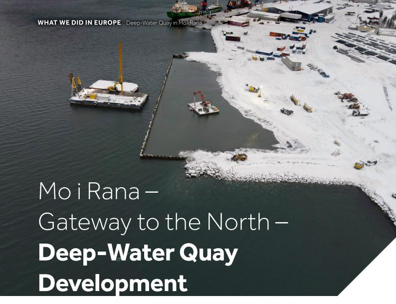
The objective of the project is to mitigate the risk of maritime accidents, enhance the capacity of port infrastructure, and improve accessibility for vessels calling at the terminals in Mo i Rana. Keller Geoteknikk AS was commissioned to carry out sheet pile wall installation, vertical drains, mass soil mixing, and piling works for the new deep-water quay development.
