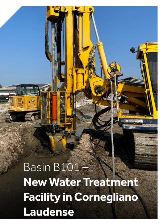
As part of the development of a new water treatment facility serving a gas storage site in Cornegliano Laudense (LO), located a few kilometres south of Milan in north-western Italy, Keller was commissioned to undertake a sensitive operation involving groundwater containment and excavation management for the construction of the underground basin 'B101'.
