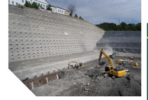
drainage boreholes and drainage mats behind the shotcrete wall prevent the build-up of water pressure.
