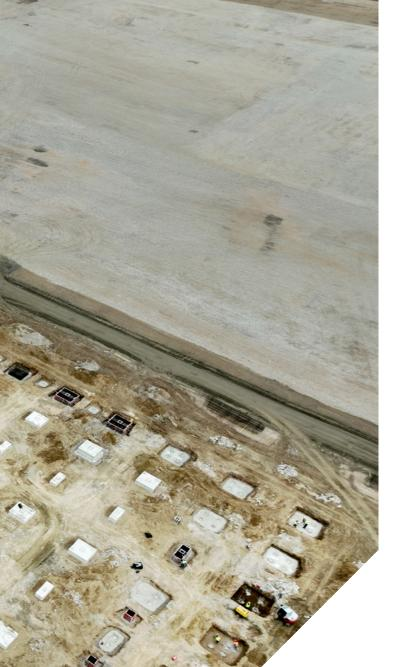
total length of piles installed was 11,707m. After the piles were completed, 332 rectangular monolithic reinforced concrete footings were constructed. The connection between footings and columns was achieved using PEIKKO anchors. The installation of these anchors had to be extremely precise to allow subsequent structural elements to be positioned correctly. The positional accuracy of individual anchors ranged from 3 to 5mm depending on the anchor type.
